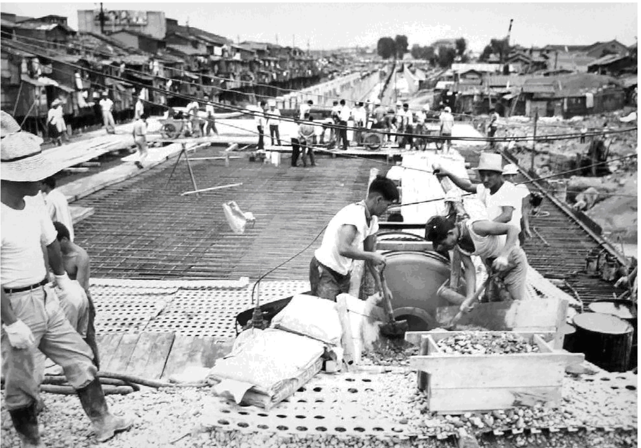
Figure 3. The Highway Construction above the Cheongcheon river in Seoul.
