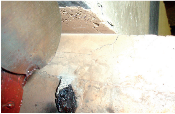
Fig. 5. Arc-shaped crack at the end of the
