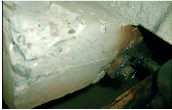
Fig. 5. Arc-shaped crack at the end of the
