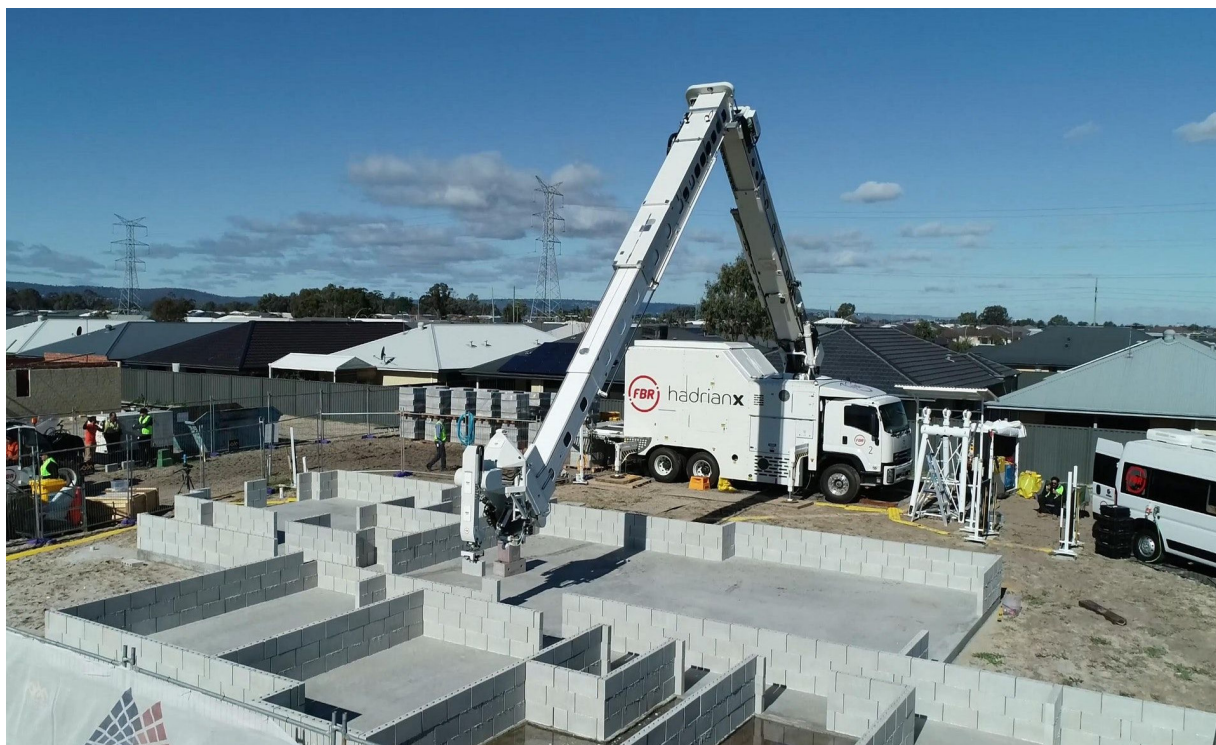
Fig. 5. Hadrian X. construction robot
