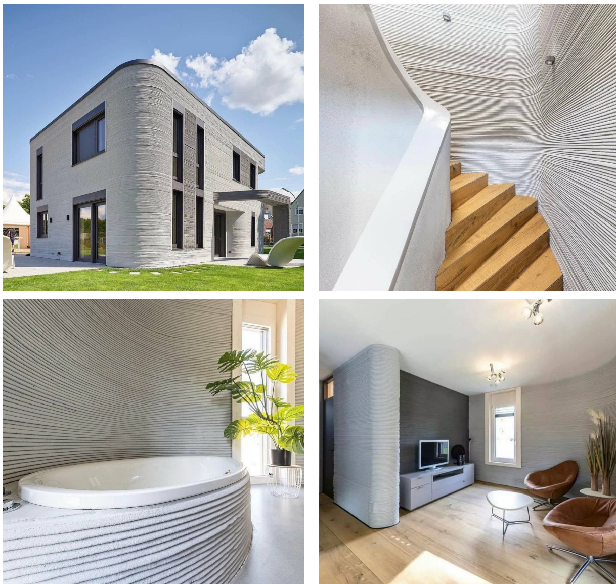
Fig. 3. The residential building construction with 3D printer, Germany
