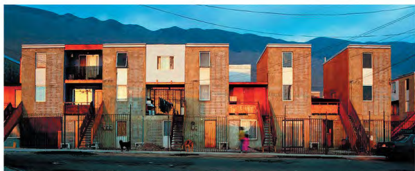
Fig. 12. Elemental Monterrey residential complex, 2009, Mexico, Santa Catarina. Architect Alejandro Aravena. Illustration of “planned self-development”: half of each house is designed, the other half is built up by residents as conditions change. The flexibility factor is realized through the combination of an ordered structure and a spontaneous one. Aravena calls the interaction of planners with the population the main principle of his work
