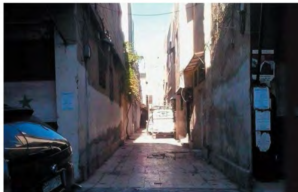
Fig. 14. One of the small roads in an unorganized residential area – Mezzeh Gardens. Damascus. Syria
