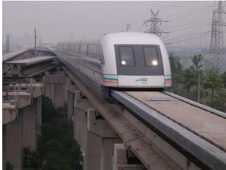
Fig. 9. EMS technology used in Transrapid (Source: Siemens AG Transportation Systems, 2005)
