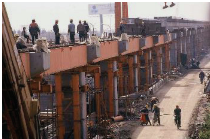
Fig. 6. Construction of Transrapid infrastructure in Shanghai [12]
