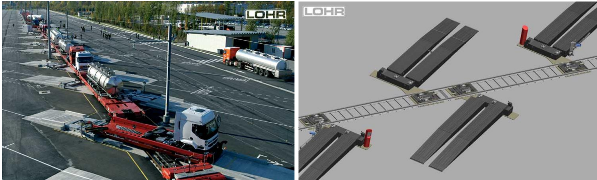
Fig. 6. The Modalohr system terminal
