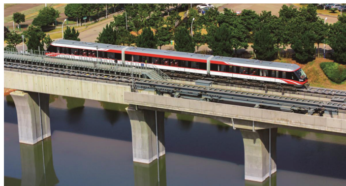
Fig. 5. Changsha Maglev vehicle running on the bridge
