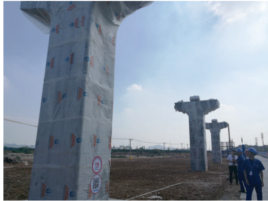
Fig. 8. Qingyuan Maglev track construction site (June 2018)
