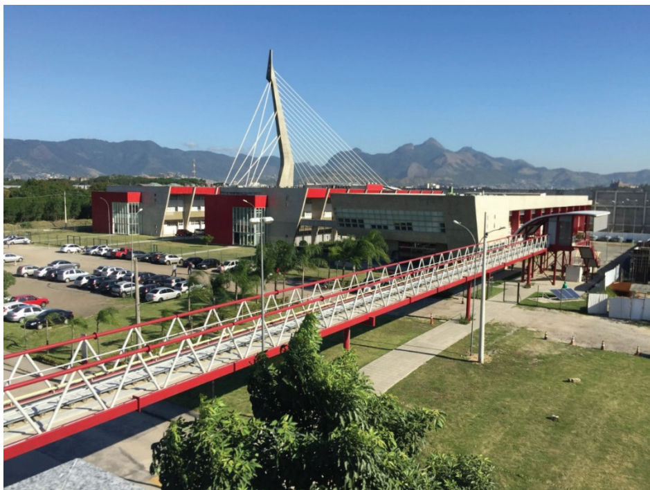
Fig. 2. The 200 meters long elevated line of MagLev-Cobra
